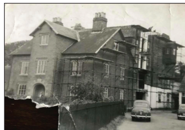
Renovations at The Rectory
